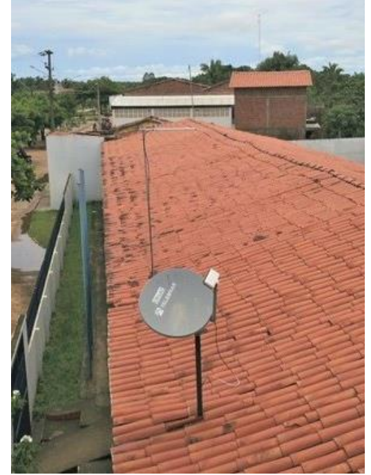
Aerial photos of satellite dishes installed at rural school facilities, utilizing Viasat infrastructure to support traffic for SGDC-1. Source: Brazil's Ministry of Communication.
