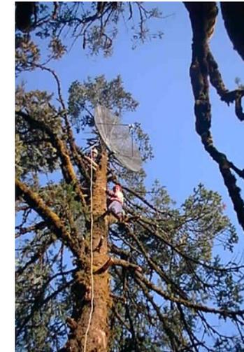
**WLL antenna fixed on a top of tree**
